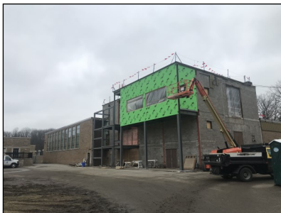
Part of the Phase 3 improvements, this space will house the new state-of-the-art laboratory at the Richard S. Wasielewski Water Treatment Plant.
