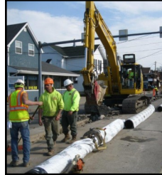
Peach Street Project
