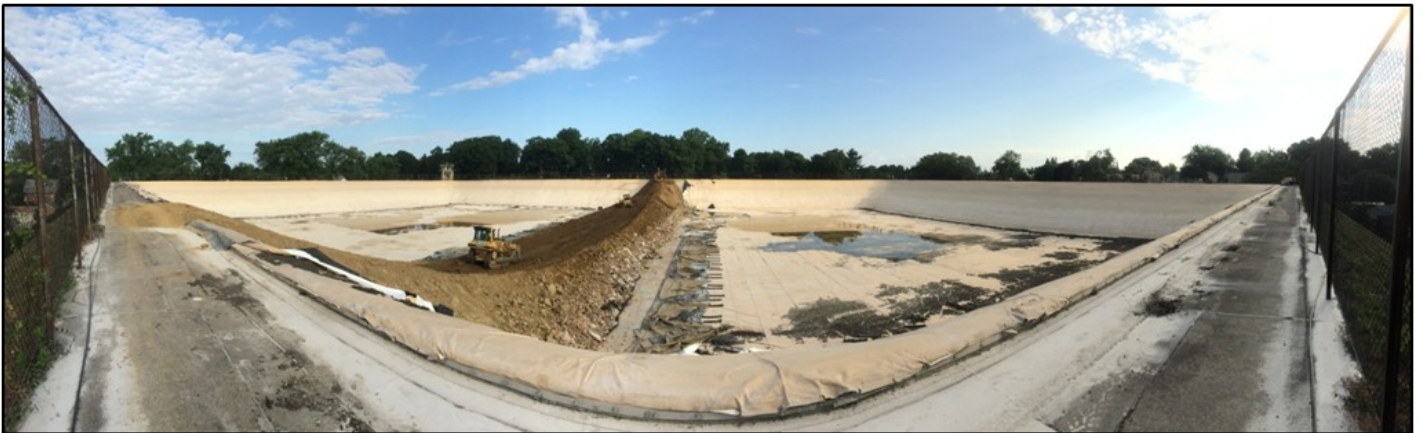
BEFORE ---> A panoramic view of the liner and 'center wall' demolition.
